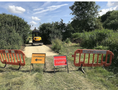
Contractors at work putting gravel down in a gateway.
