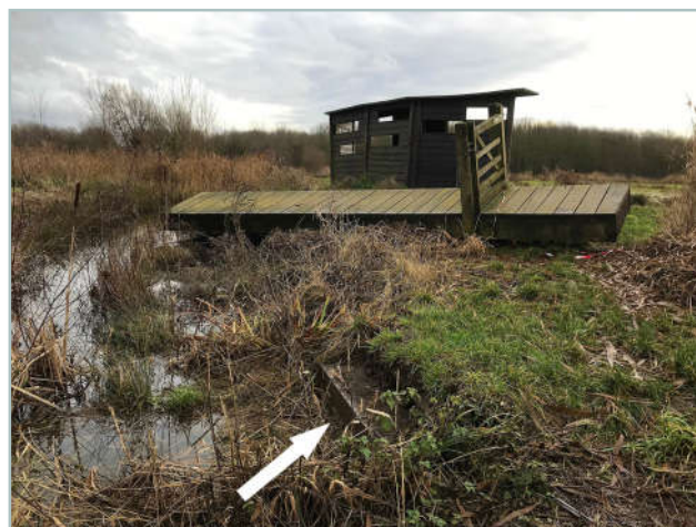
The scrape bridge floated away in the flood. The white arrow shows where it came from! Photo: Richard Stott
